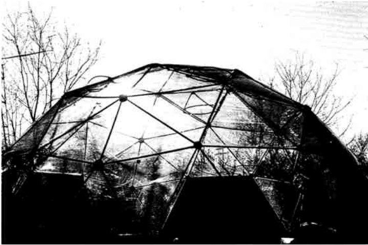
FIGURE 39-5 Prototype bioshelter. A geodesic dome housing fish and vegetable modules. Photo by J.Todd.
