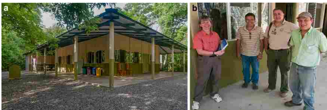
Fig. 5 a Newly constructed research house in Sector Santa Rosa, Área de Conservación Guanacaste (ACG), 2011. b Left to right Linda Fedigan, Marvin Jimenez Salas (contractor/builder), Roger Blanco
